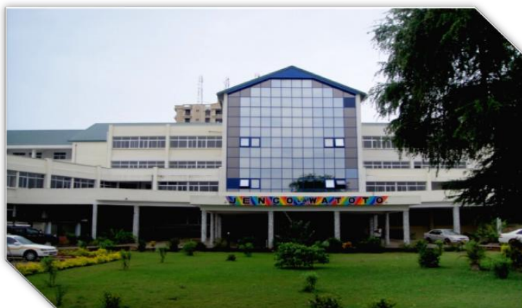
The New Paediatric Building at MNH
